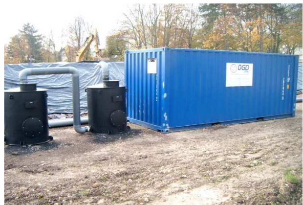
Connection and covering of the biopile
