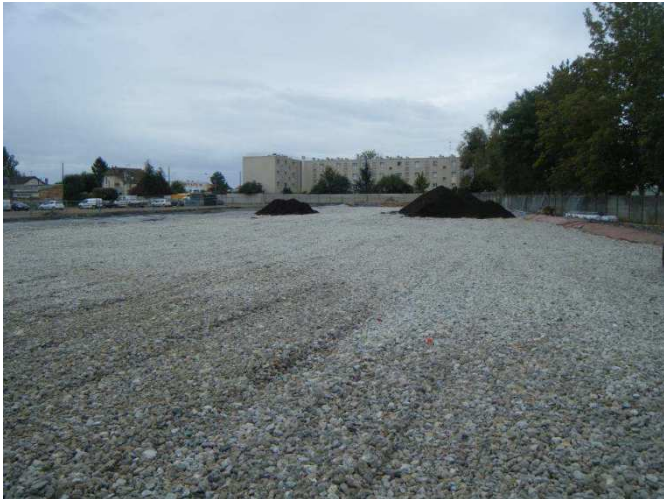
Creation of the waterproof platform with drainage layer
