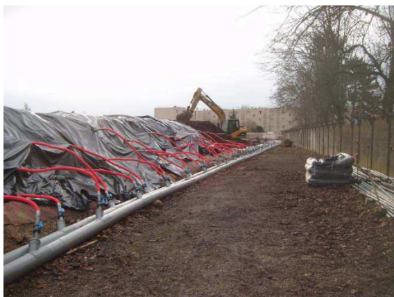
Connection and covering of the biopile
